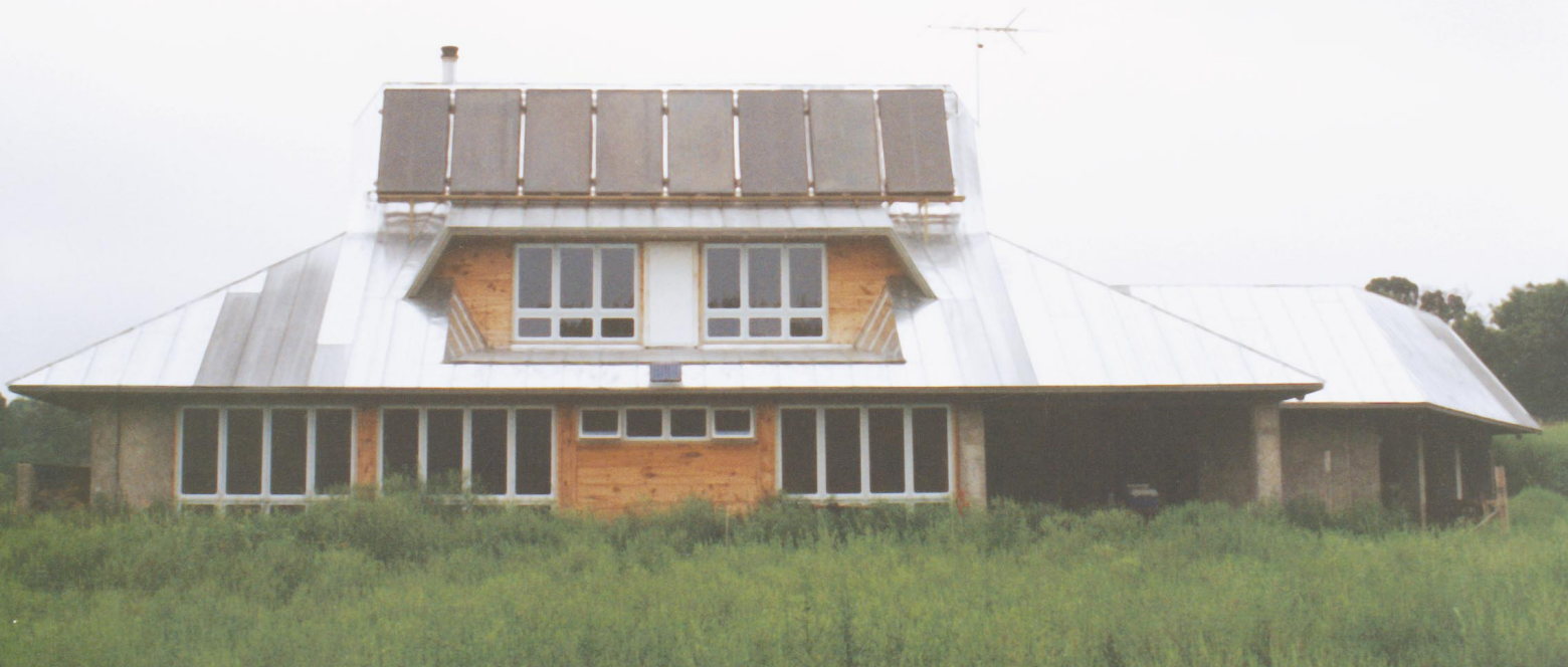
Above: The south-facing Haasch house is solar-hydronic heated.
